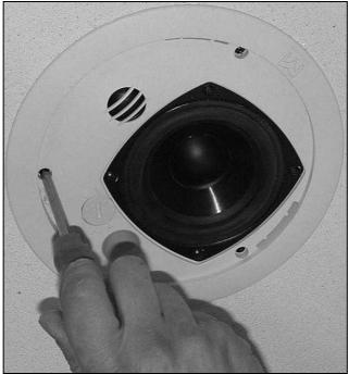
**Tightening the swivel-tab screws**
